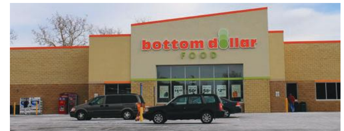
Figure 7.78 - A new grocery store constructed in 2012.
