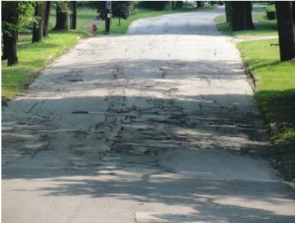
Figure 4.2 - Road conditions on Volney Road.
