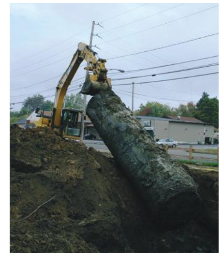
Figures 5.18-19 - Underground Storage Tank removal in 2012 along Glenwood Avenue.
