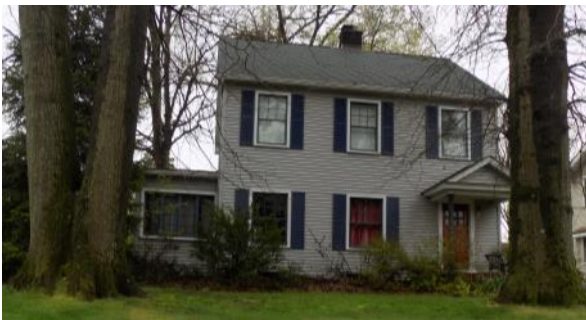
1543 CANFIELD: BEFORE REHABILITATION
