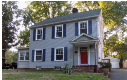
1543 CANFIELD: AFTER REHABILITATION
