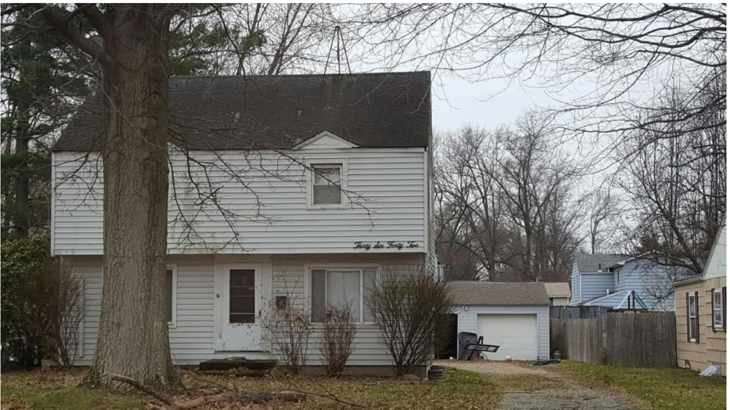
A blighted, vacant structure on Arden Blvd. has a detrimental effect on surrounding properties
