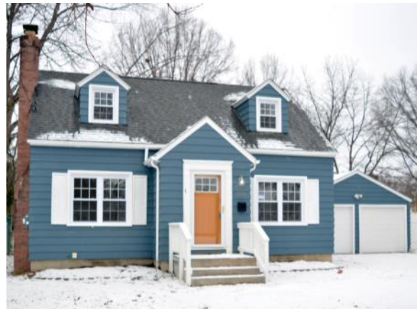
2136 GREGORY: AFTER REHABILITATION
