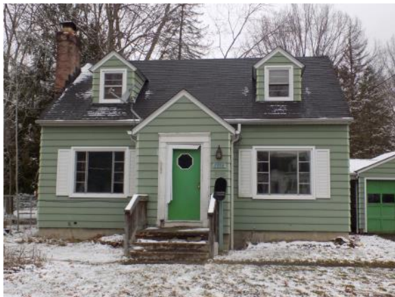
2136 GREGORY: BEFORE REHABILITATION
